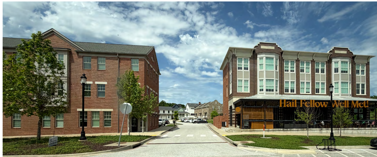
The development pattern of Johnson Square could be replicated in other parts of the city.
