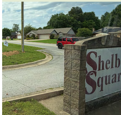
The commercial center in the foreground sits across Main Drive from several single family homes.
