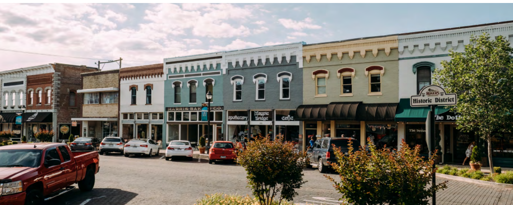
This historic district in Rogers features a classic main street commercial area.
