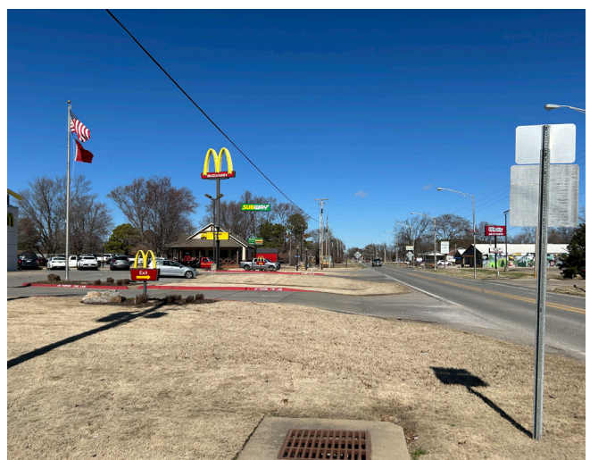
Sidewalks would be a welcome addition to this commercial area.
