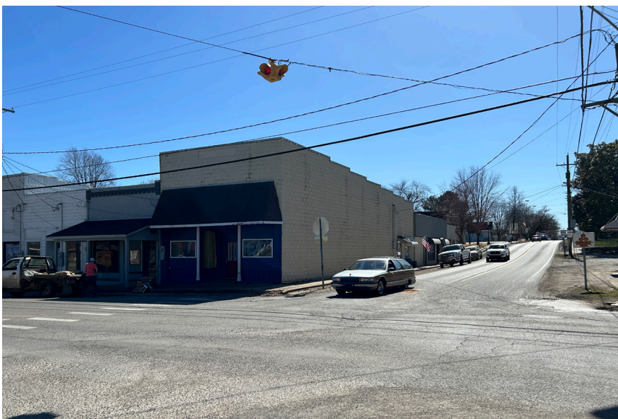
The infrastructure in the city's historic downtown creates an environment for pursuing infill development.
