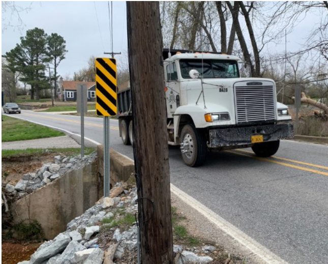
The culvert at the northern edge of downtown creates tight passage for vehicular traffic, with no room for pedestrians or bicyclists.
