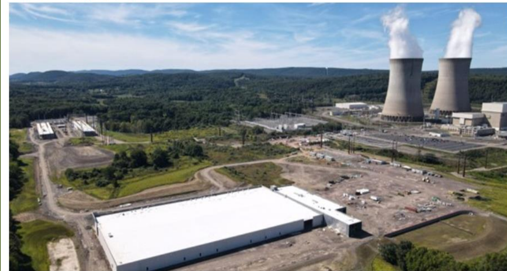
Susquehanna nuclear plant in Salem Township, Penn., along with the data center in foreground. (Photo: Talen Energy)
