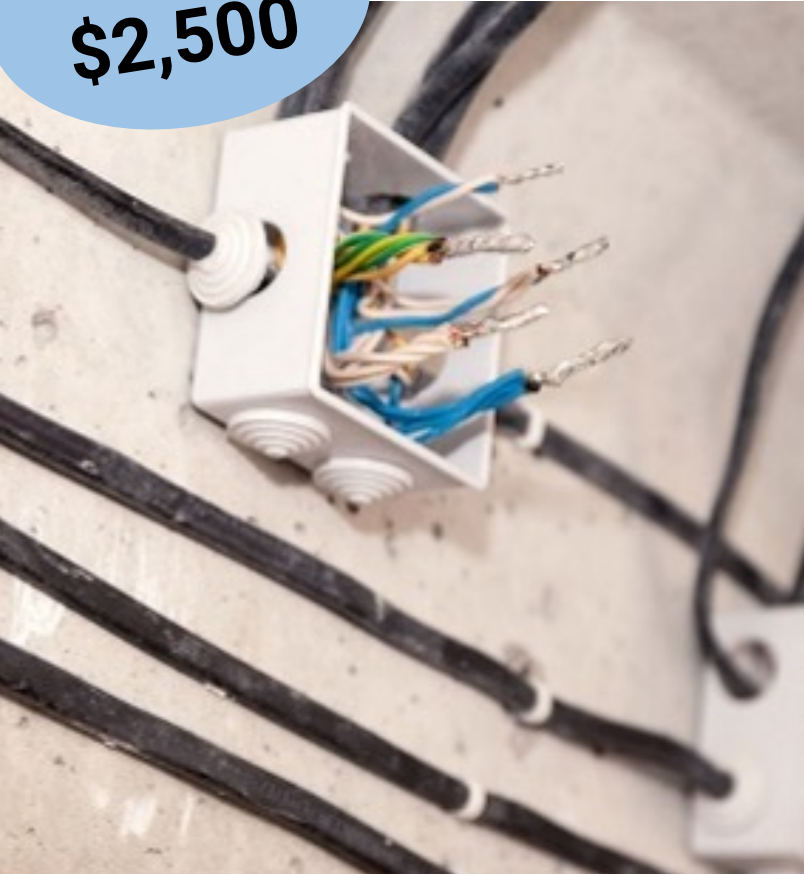
Electric Wiring Upgrade
