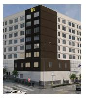
An adaptive reuse project is transforming an existing student housing building known as "The G" into a tru by Hilton with 185 rooms. The building will be stripped down to the concrete shell and rebuilt with new exteriors, interiors, and a third elevator. The top floor of the parking garage will be converted into lobby space with a bar, lounge, gym, and reception. Completion is projected for March 2026, welcoming UT visitors, parents, and fans.
