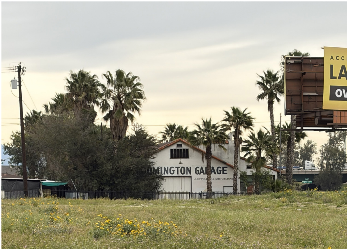
The historic Bloomington Garage currently is hidden in the back of an underdeveloped lot along Valley Blvd.
