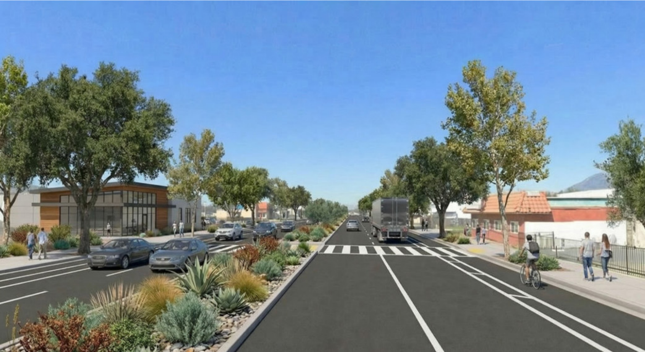
A visual of updated streetcape investment along Valley Blvd., with repaired and resurfaced roadway, landscaped median, underground utilities, continuous sidewalks and street trees, and a buffered bike lane.
