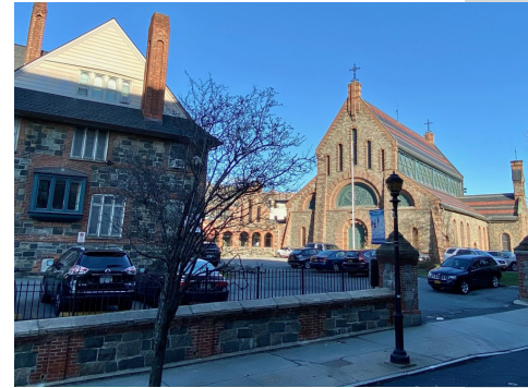
St. John's Episcopal Church at Getty Square, view from the south. Source: TAP Panel.
