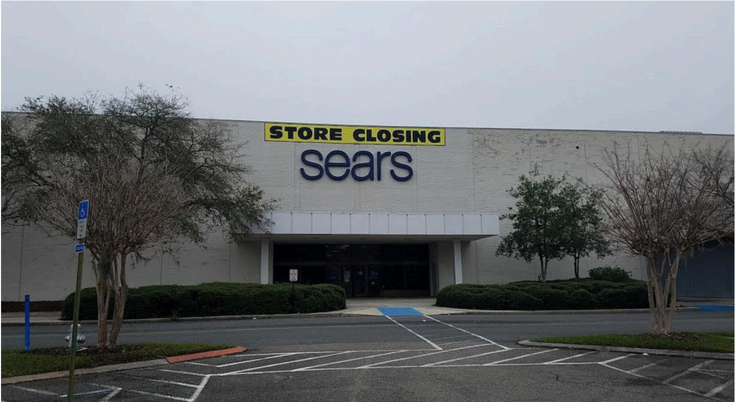
PHOTO: Abandoned Sears property
