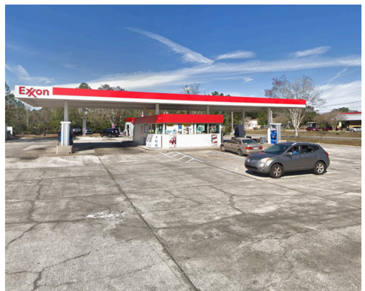
PHOTO: Gas station on Blanding Boulevard
