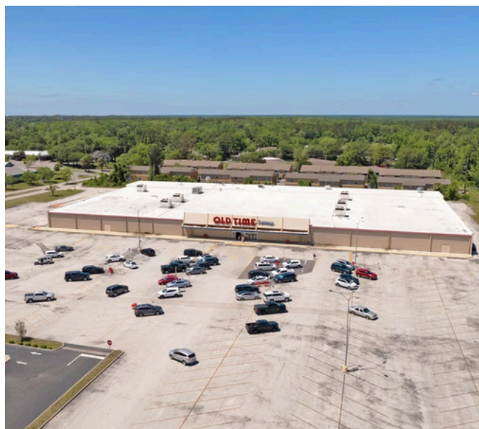
PHOTO: The 9-acre site occupied by Old Time Pottery could be ripe for redevelopment.
