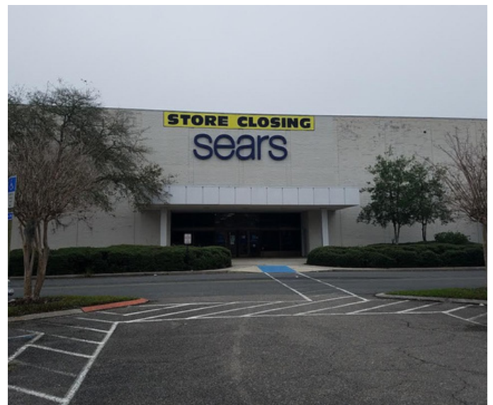
PHOTO: Abandoned Sears property
