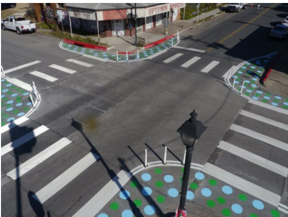
PHOTO: Example of painted bulb-outs, Austin, TX
