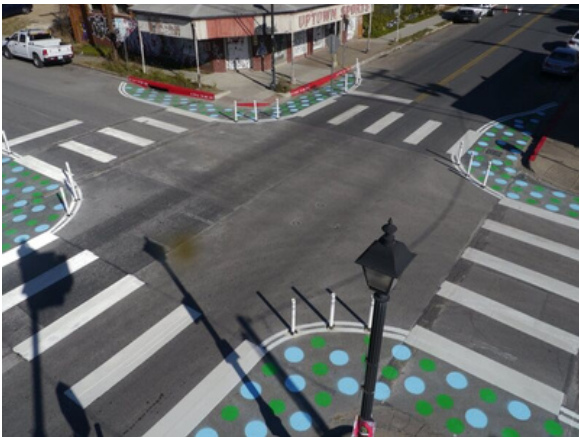
PHOTO: Example of painted bulb-outs, Austin, TX
