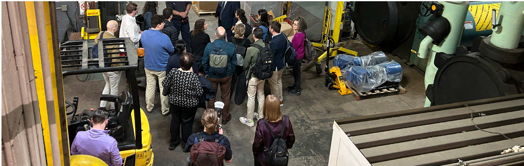
The Penn South cogen facility runs on a combination of natural gas and diesel, powering 2,820 apartments.
