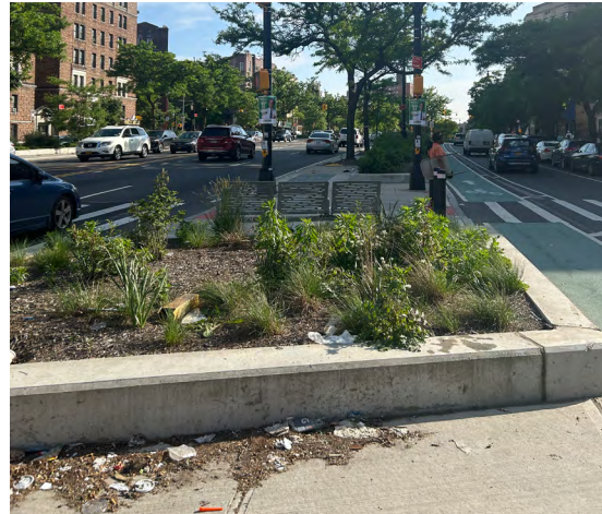
The median along Grand Concourse is well-planted, yet litter and debris continue to collect on the edges.
