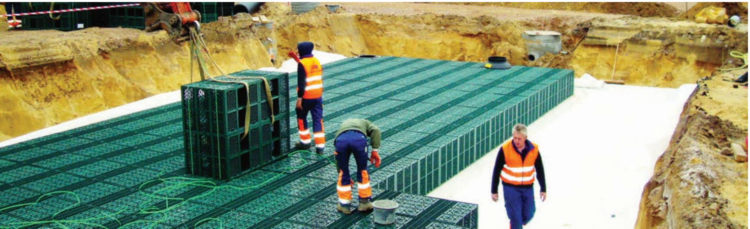
IMAGE CREDIT: Infiltration Crates | Rainproof Amsterdam | www.indra-infra.com
