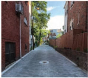
Alley Permeable Pavement (APP), also known as green alley
