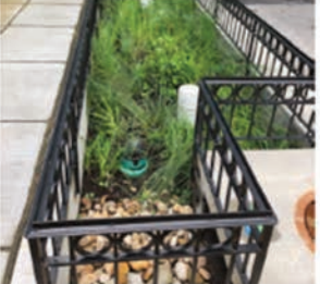
Planter Bioretention (PBR)
