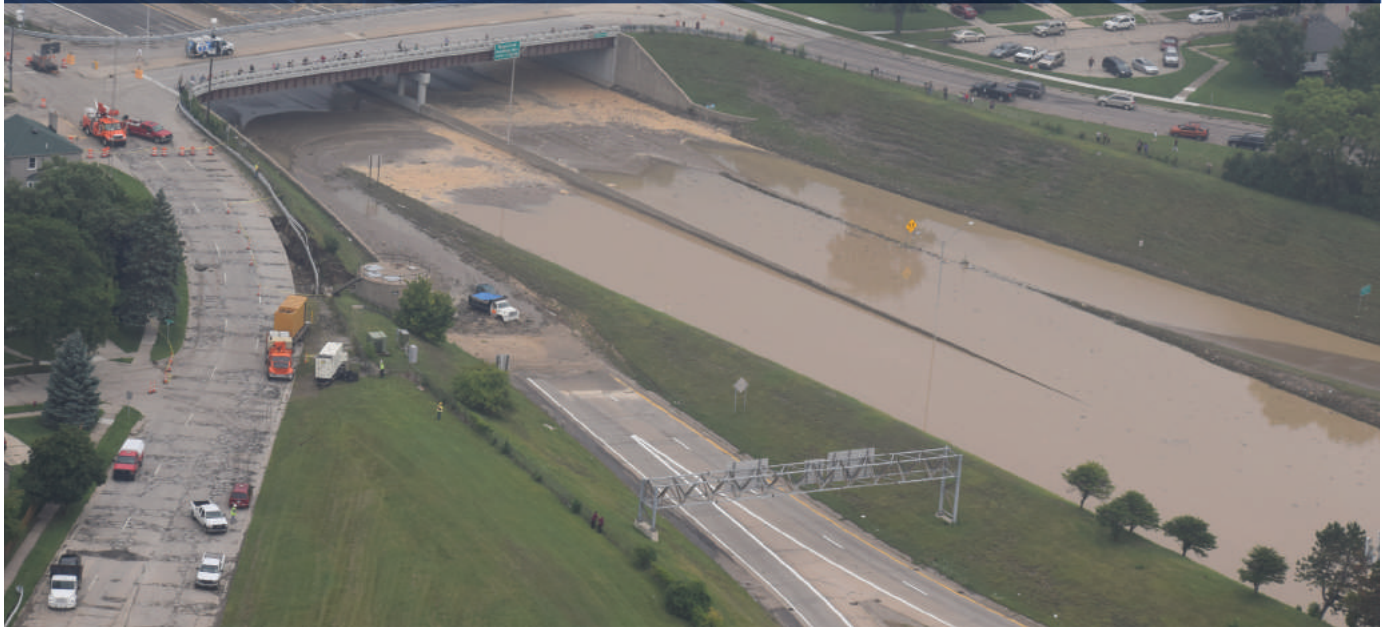
Highway flooding and embankment collapse, August 2014 (Michigan State Police Emergency Management and Homeland Security Division)
