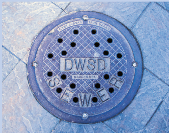
Detroit Water and Sewerage Department Sewer Cap (Michael Kumm)
