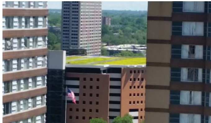
Coleman A. Young Municipal Center Green Roof (Trisha White)
