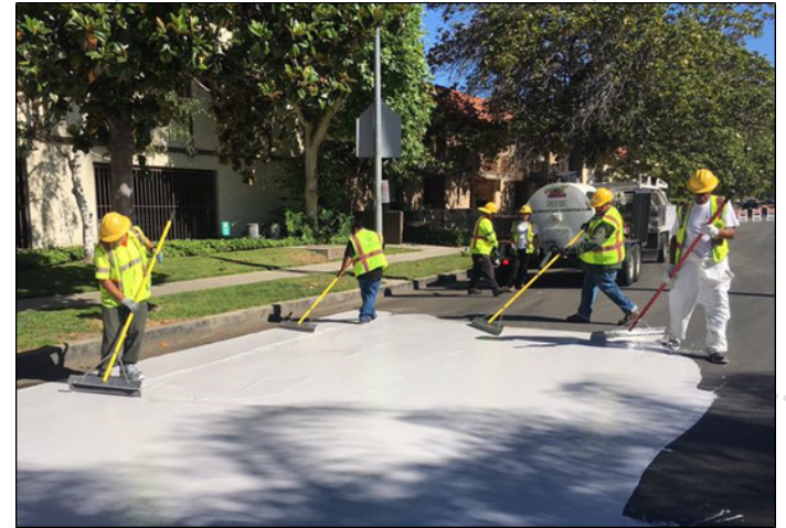
Cool Seal product being installed in Los Angeles
