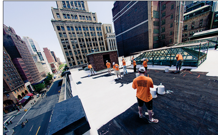
A "cool roof" being installed on an existing building in New York City
