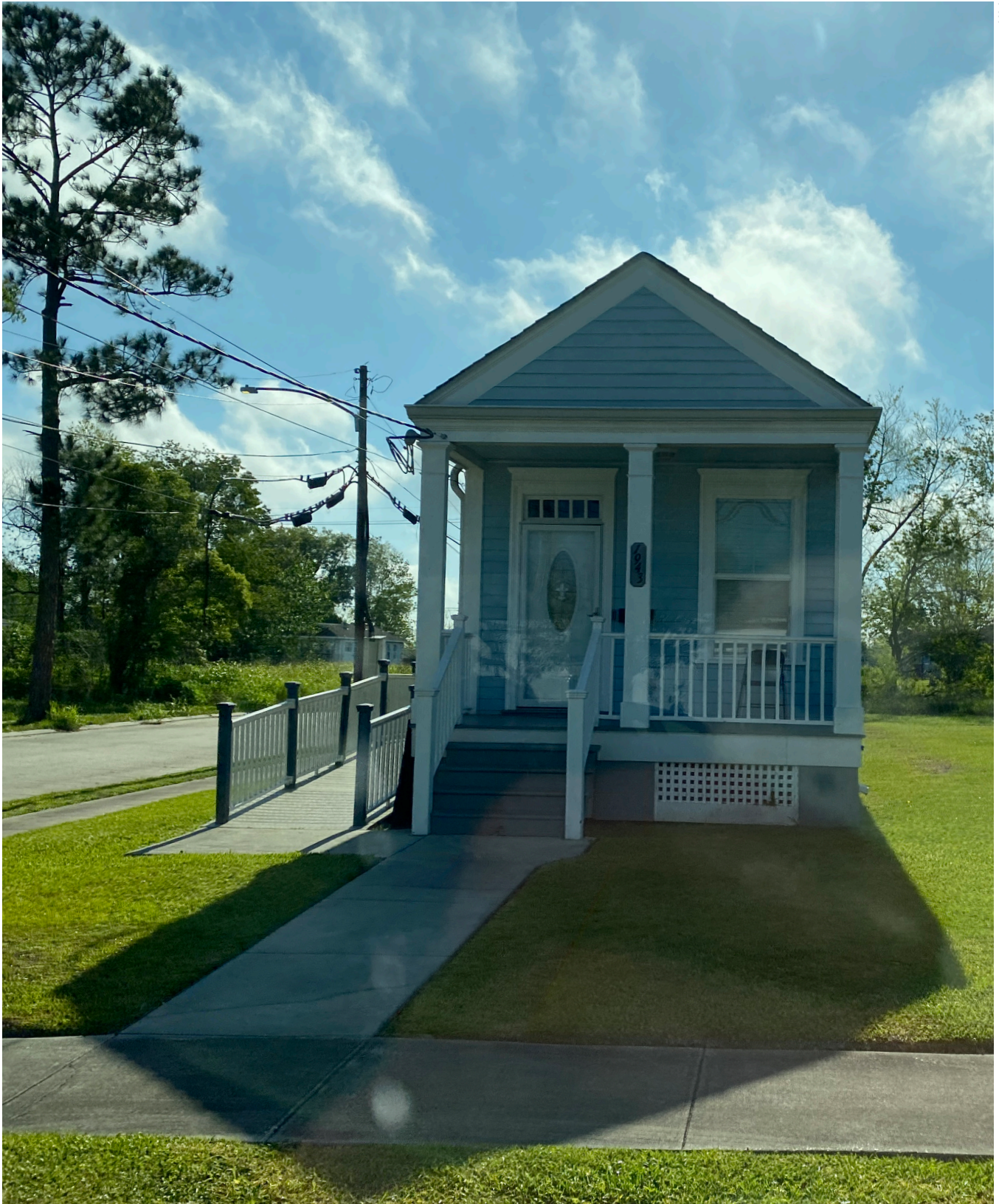
Housing conditions in the Lower Ninth Ward vary wildly from neatly maintained, as seen in this home along Tricou Street, to needing significant repair.
