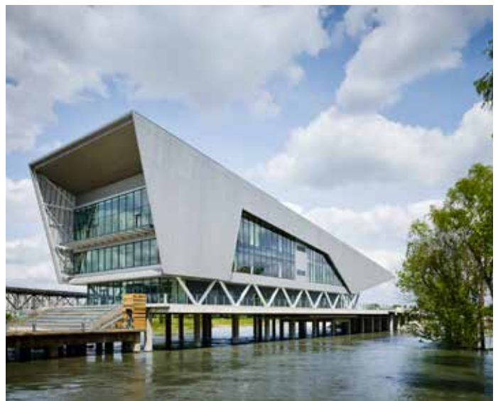
The Water Campus, Baton Rouge
