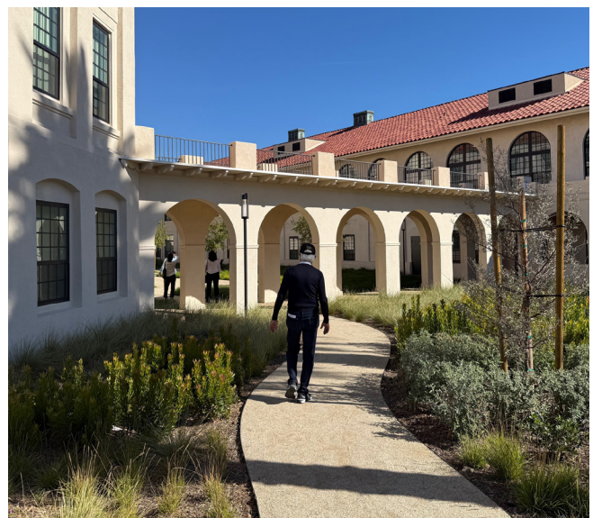
The development of student veteran housing as a component of supportive housing on-site represents an opportunity for homelessness prevention while encouraging educational and technical goals.
