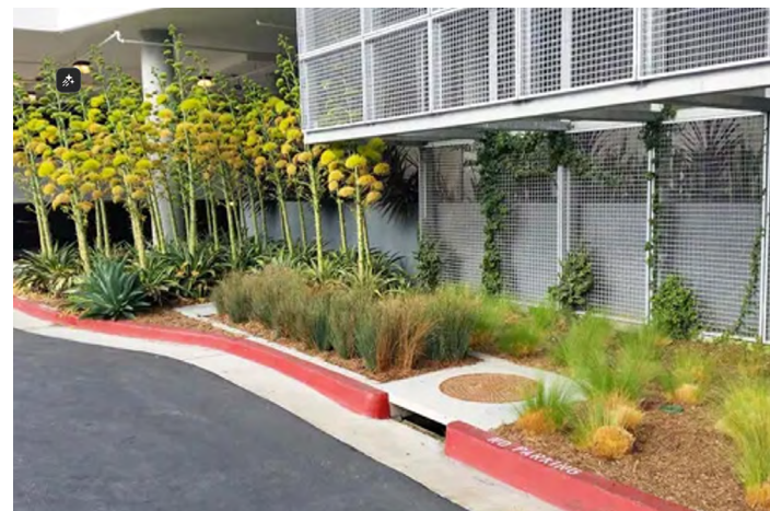
This stormwater drain is assisted by the surrounding rain garden and native plants, designed to capture and reuse rainfall.
