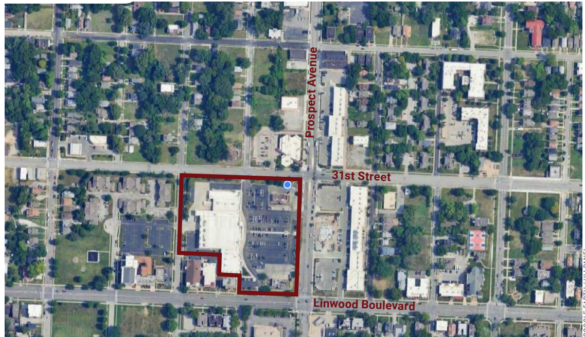
The Linwood Shopping Center, home to the Sun Fresh Market, is outlined in red.
