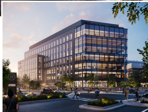
ISQ 3 (Currently under construction)
