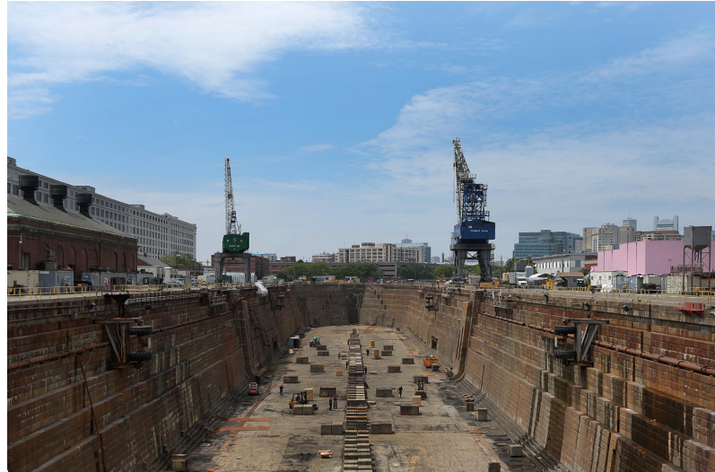
MARINE INDUSTRIAL PARK Boston, Massachusetts
