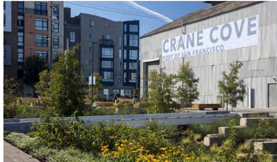
ABOVE TOP Aerial view of Crane Cove Park Image credit: AECOM
