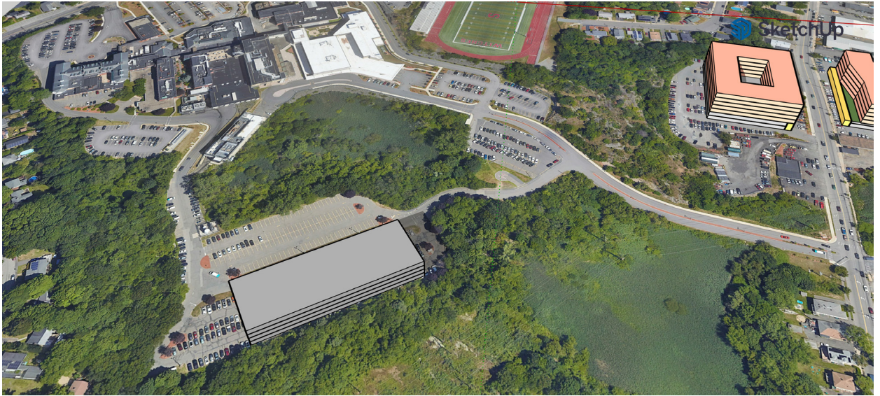
This sketch considers how a four-level garage could be placed to accommodate the redevelopment of the Jefferson West lot.
