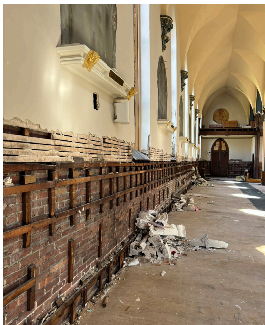
The plaster walls in the sanctuary need significant repair.
