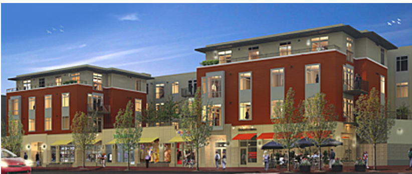
Zone 1 - 29 Albany Street / Central Garage.
