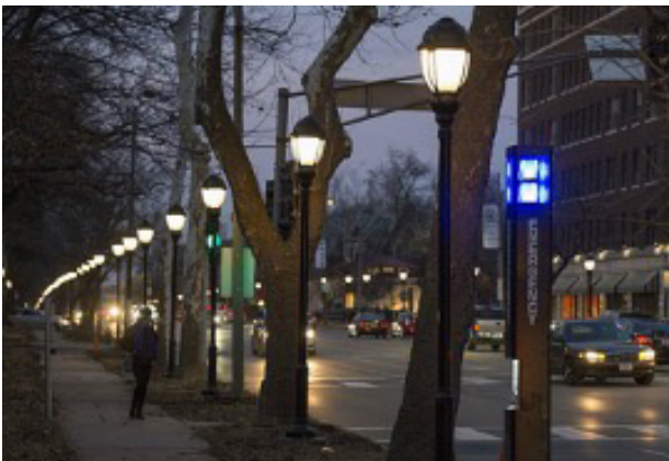
New sidewalks, safety lighting, paving E. Worcester/Albany.
