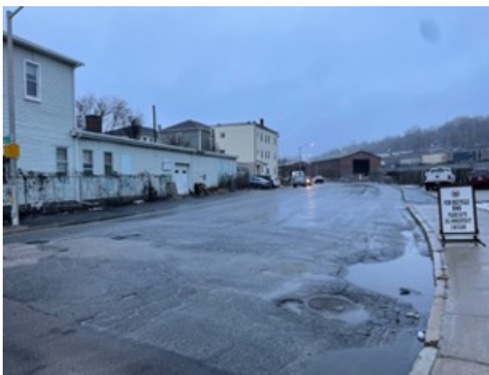
Existing conditions along East Worcester Street.
