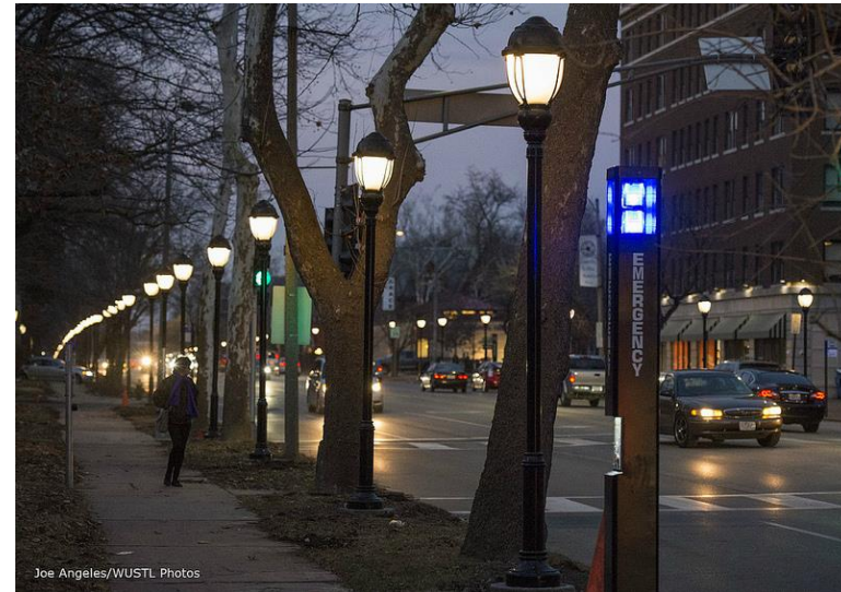
New Sidewalks, Safety Lighting, Paving E. Worcester/Albany
