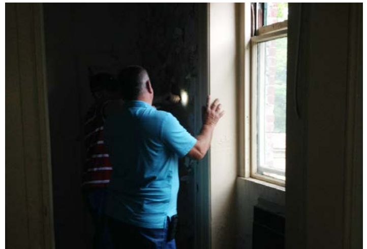
Panelists examine the condition of the Administration Building.
