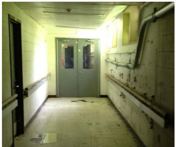
Interior of the Daniels Office Building
