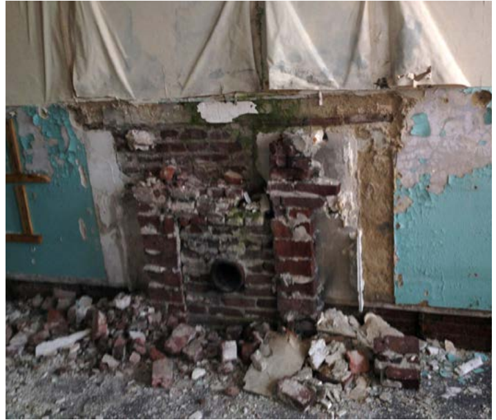
Interior of the Administration Building
