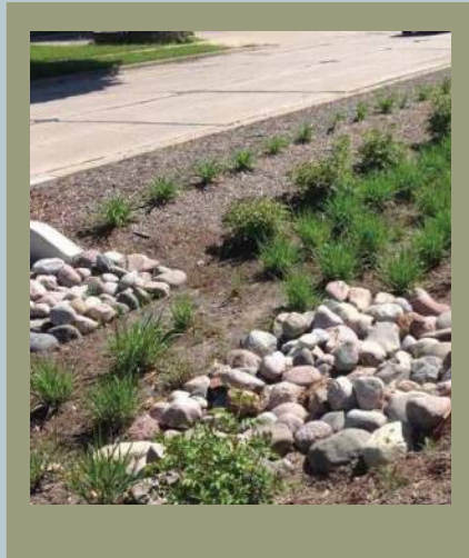
Bioswales + Pervious paving
