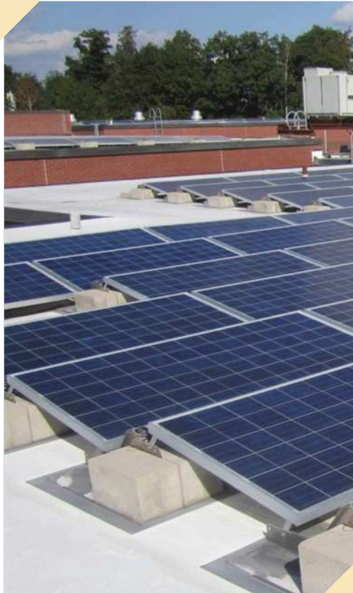
Solar-ready roof structure
