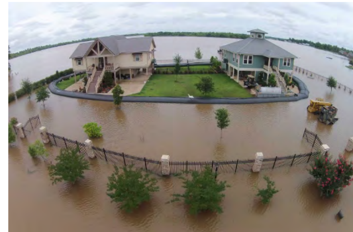
Water-filled flood protection tubes can be used to protect buildings from flood waters.
