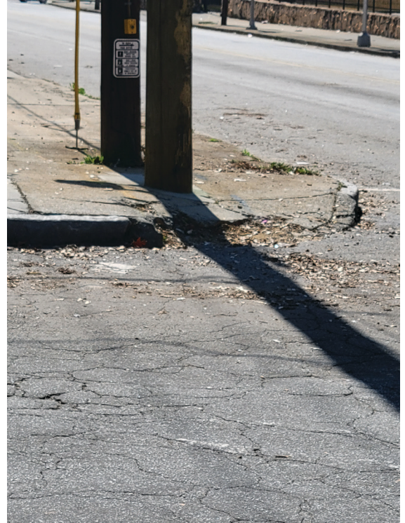
Crumbling sidewalk ramps need repair or replacement.
