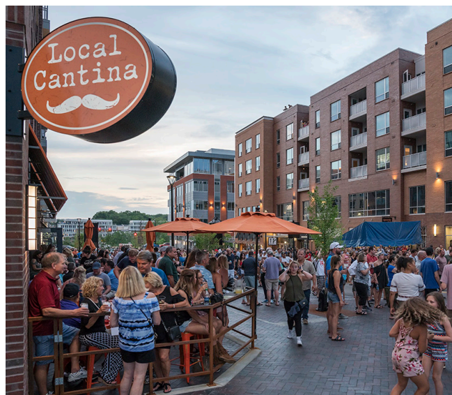
In Dublin, Ohio, the 30-acre Bridge Park is a good example of a walkable, mixed-use community built close to transportation resources while remaining focused on the pedestrian experience.
