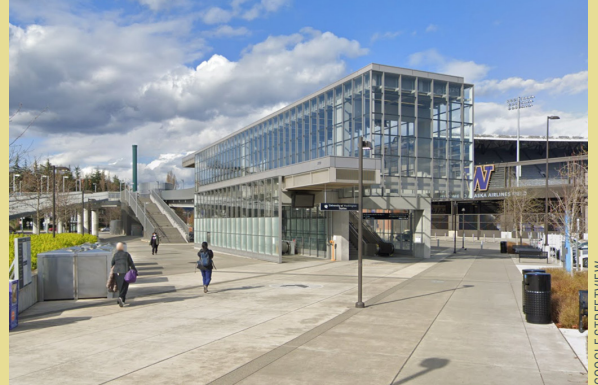
The University of Washington Sound Transit Station in Seattle, Washington, provides good connectivity across modalities.
