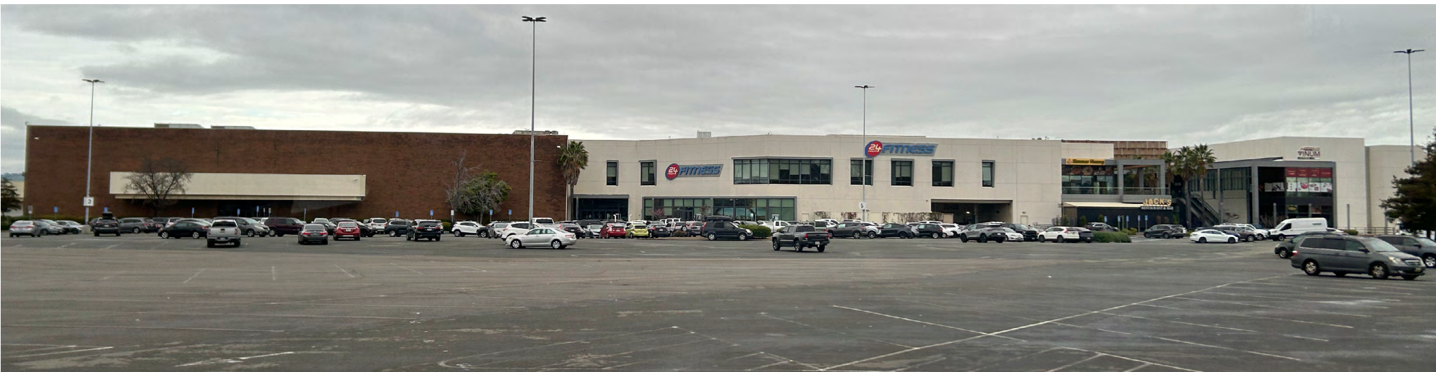
A 24-Hour Fitness facility has filled a section of the mall that is visible and directly accessible from the surrounding parking lots.
