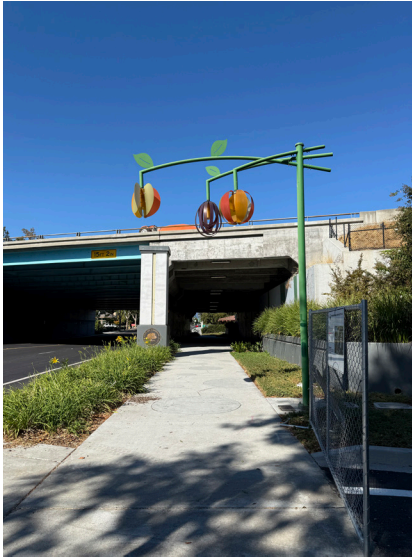
East Campbell Avenue Bridge - Portals Project
