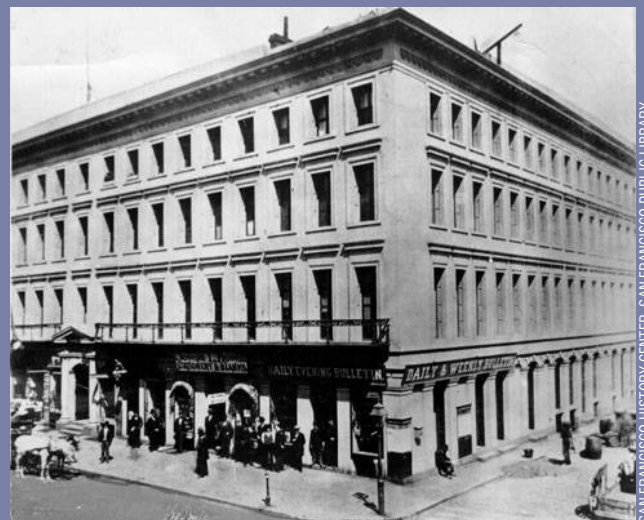
The Montgomery Block building in 1880.
