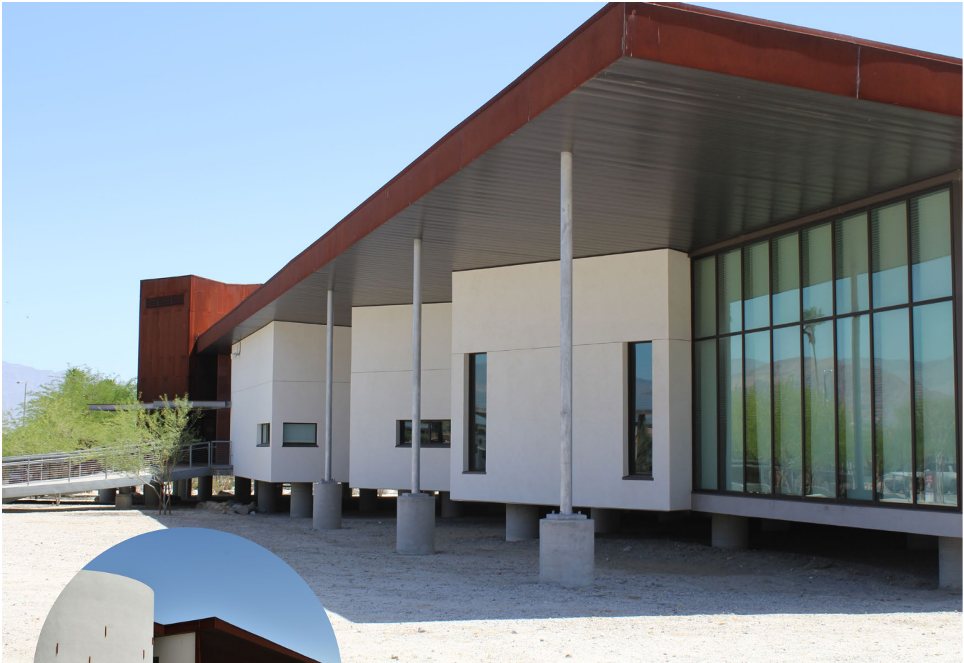
The library, adjacent to the project site, is elevated due to the flood zone.
