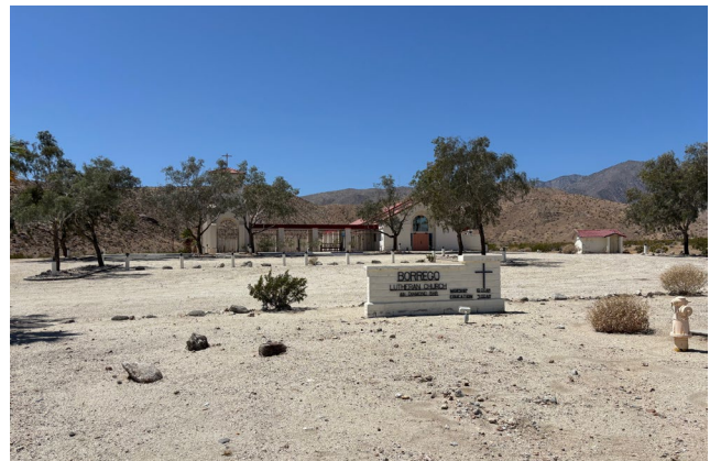
The Borrego Lutheran Church is adjacent to the project site.
