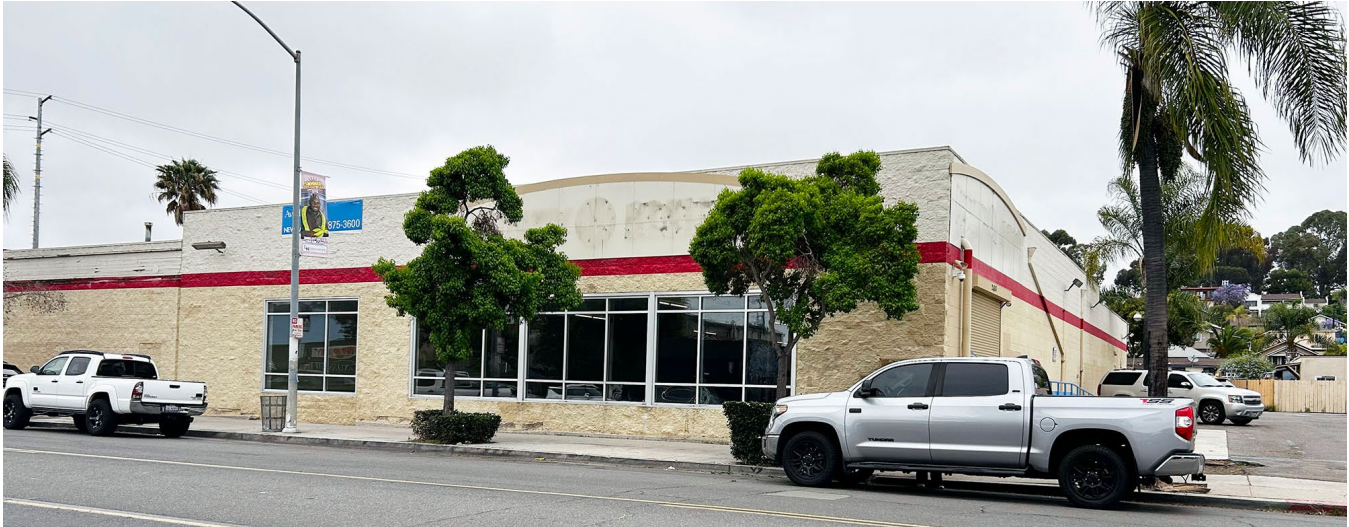
Vacant big-box retail space.
