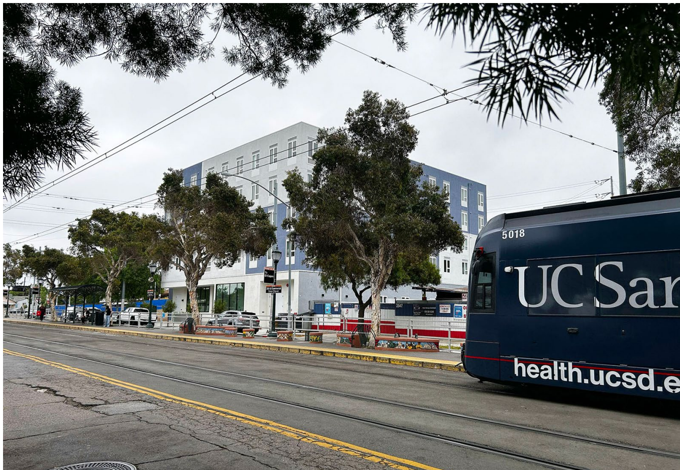
New multifamily housing at trolley station.
