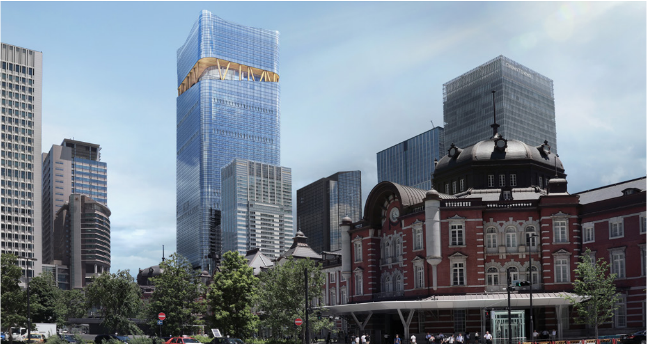
Perspective of Torch Tower seen from Marunouchi side of Tokyo Station
