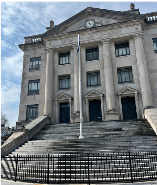
The Upper Darby Township Municipal Building.
