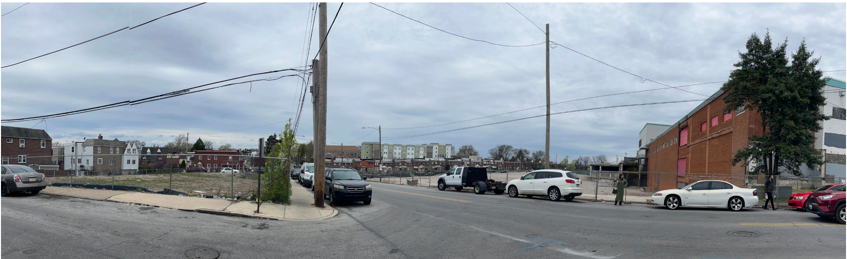
View of Walnut Street with the vacant lot of the former Upper Darby Multi-purpose Center on the left and on the right the vacant lot where the former Sear's building parking garage was. Both sites were presented to the panel as options for creating open space or potential development sites.
