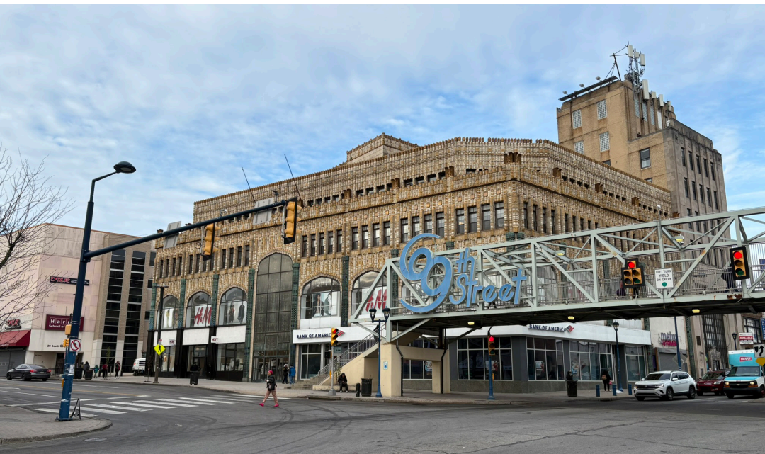
View of the pedestrian bridge with 2 S. 69th Street in the background.
