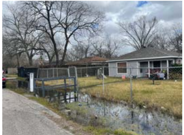
Figure 24. A flooded open drainage ditch filled with trash in Settegast. The flooding is preventing access to this home. Source: HCPH. (2022).
