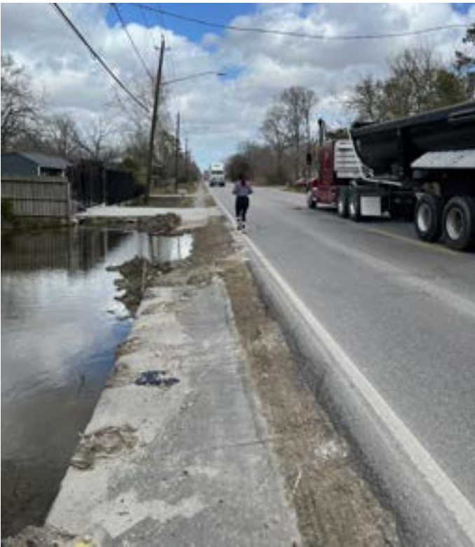
Figure 23. A damaged sidewalk forces a woman to run in the road next to 18-wheeler trucks. Source: HCPH. (2022).
