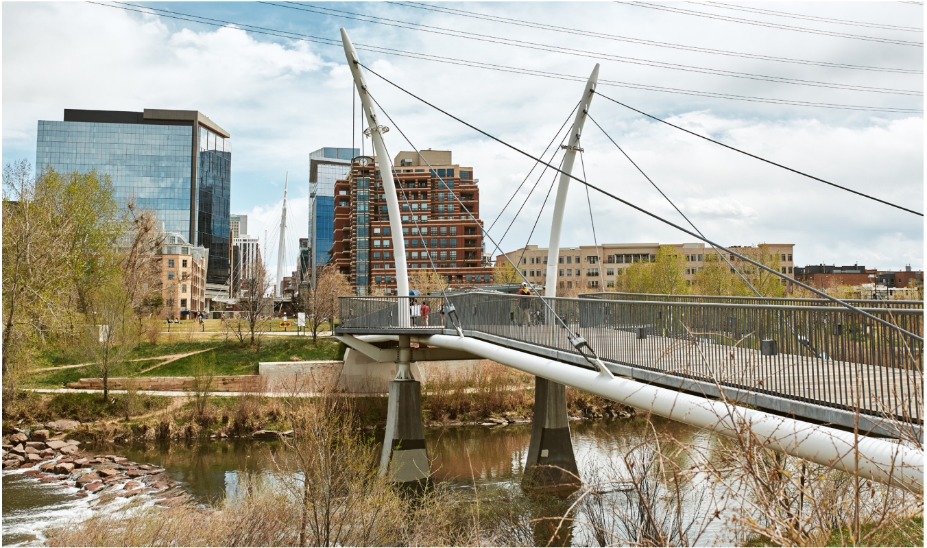
The South Platte River Bridge in Denver's Commons Park connects the Lower Downtown neighborhood with recreation opportunities and alternative modes for commuting to downtown Denver.
