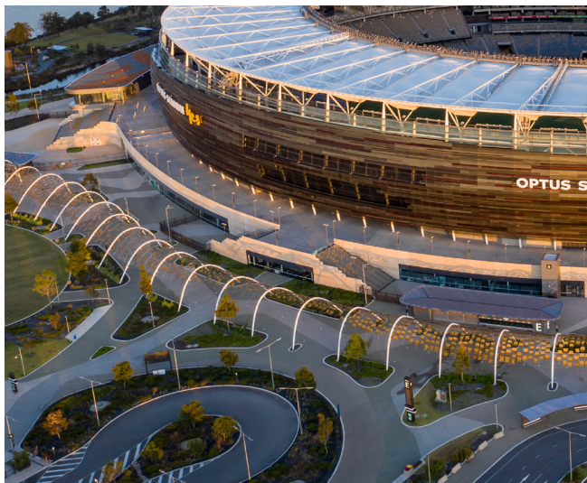
The pedestrian experience around this stadium is artful, engaging, and fully separate from automobile traffic.
