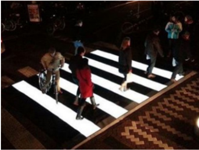
Innovative crosswalks, such as this one featuring lighted stripes, create a defined pedestrian space and further enhance safety.
