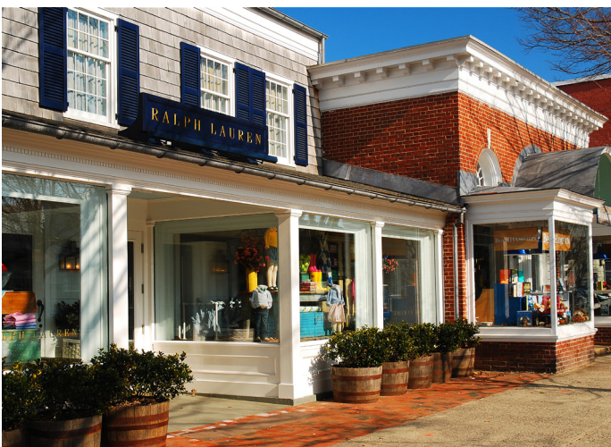
Streetscapes featuring one-story retail can be just as inviting and interesting as multistory streetscapes.
