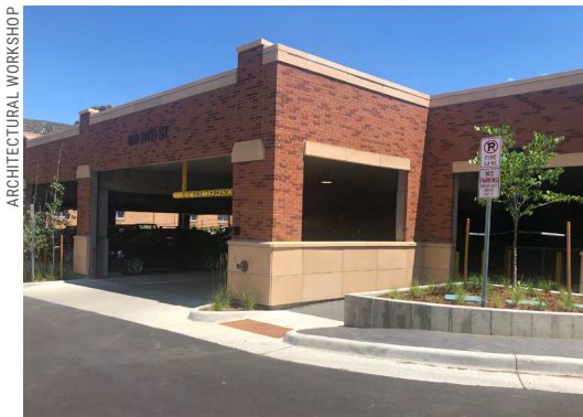
This garage in Golden, Colorado, serves a nearby church congregation, provides public parking for a fee, and also serves as festival space for the community.
