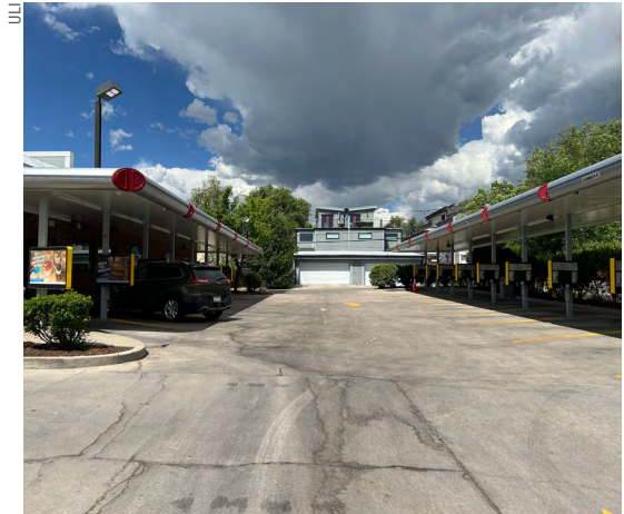
A view of the Sonic drive-thru lane to the alley beyond.
