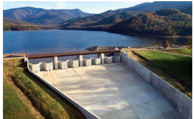
The North Fork Water Treatment Plant was hit hard by Tropical Storm Helene. Establishing a fourth water treatment plant will help alleviate strain on the system and help mitigate the effects of future storms.
