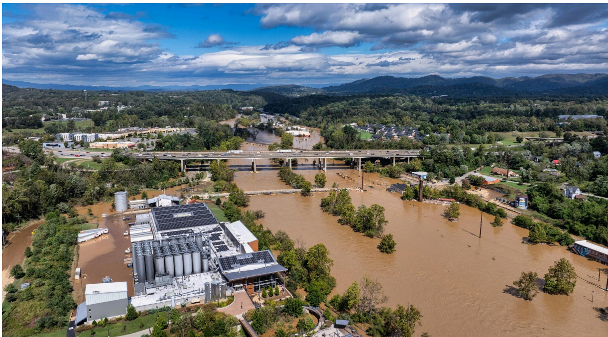
Flooding of French Broad River in Asheville NC / Courtesy of Reggie Tigwell Curve Theory
