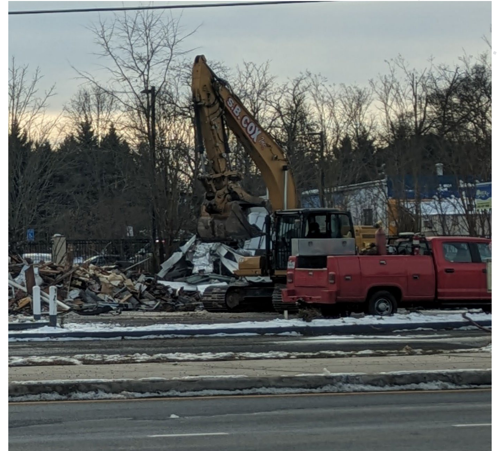
Demolition of gas station at 8851 Richmond Highway/ Credit: ULI
