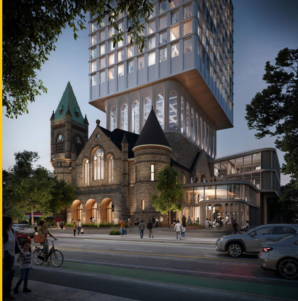
St. Luke's United Church 355 Sherbourne Street
