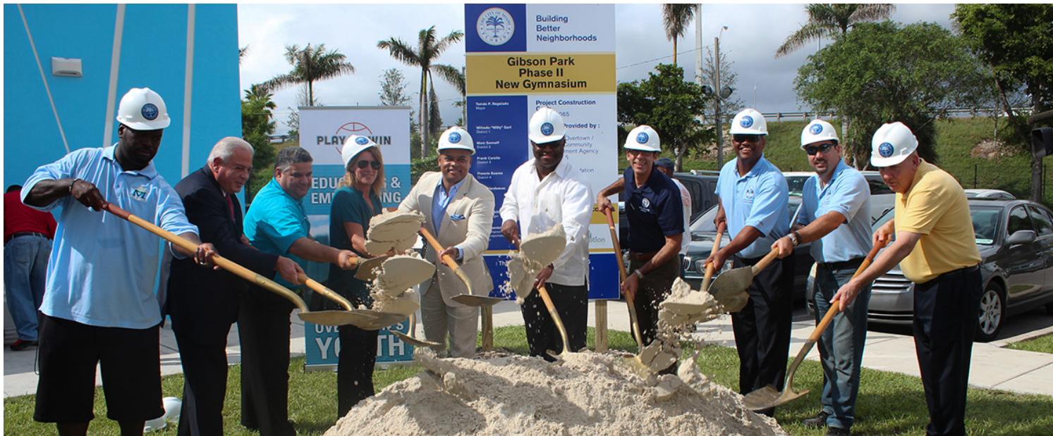
Above: Groundbreaking at the City of Miami’s Gibson Park Phase II Redevelopment project. Grants and funding mechanisms can support redevelopment efforts like these in Deerfield Beach.
