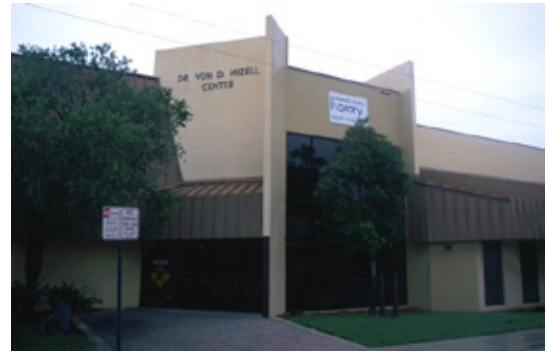
Figure 7: The Mizell Center, Segment 2.
